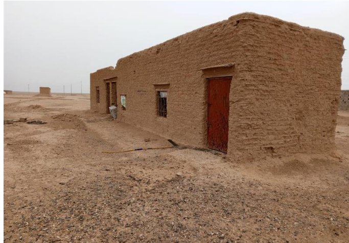
Figure 2 A mud house in the village, built with traditional materials and simple construction
